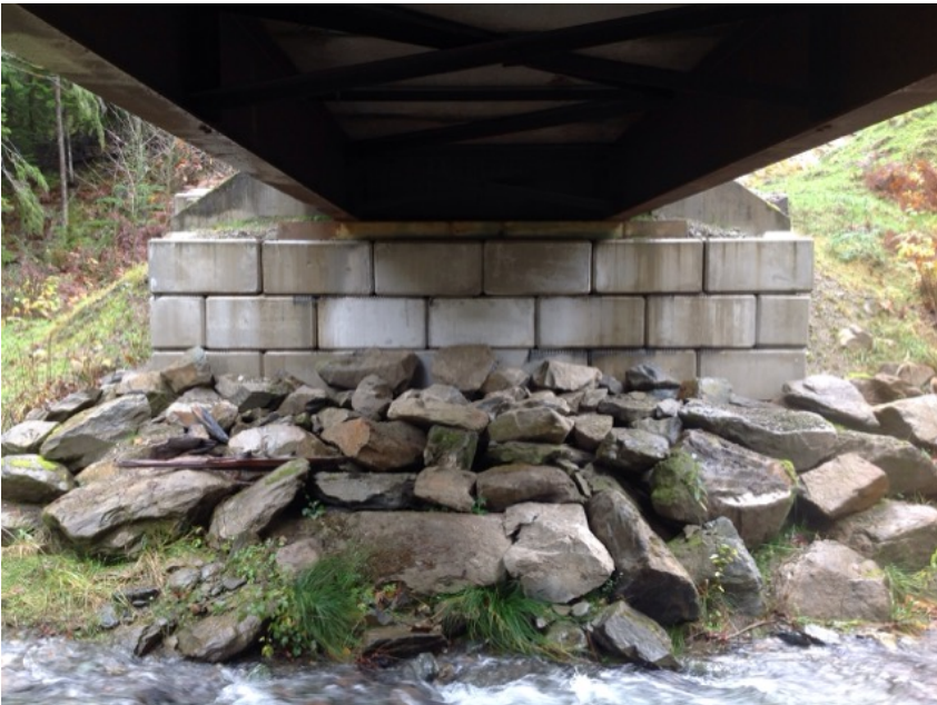
Left Bank Abutment when facing downstream
