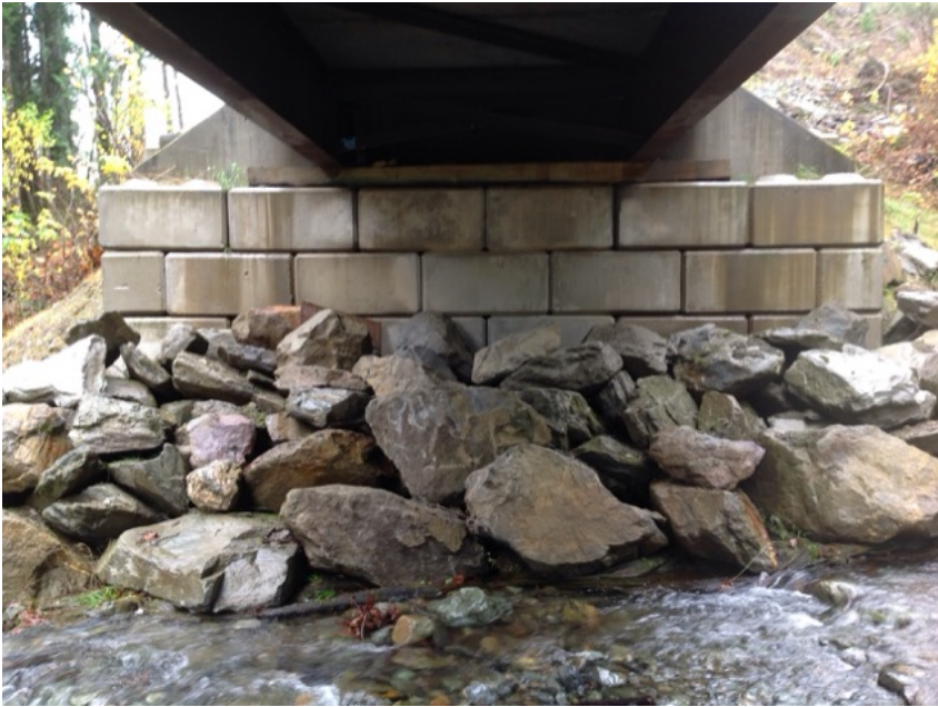
Right Bank Abutment when facing downstream
